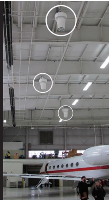
Recent Airius installation (Air Pear fans circled) in corporate jet hangar.
