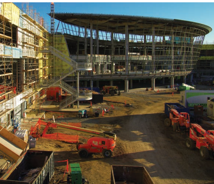
San Diego International Airport expansion.
