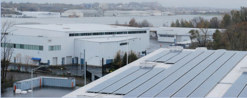
Hurricane Sandy-damaged Teterboro Airport.
