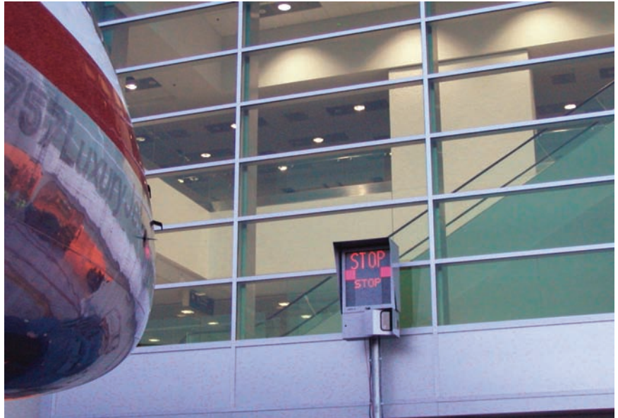
American Airlines parks using A-VDGS at Miami International Airport.
